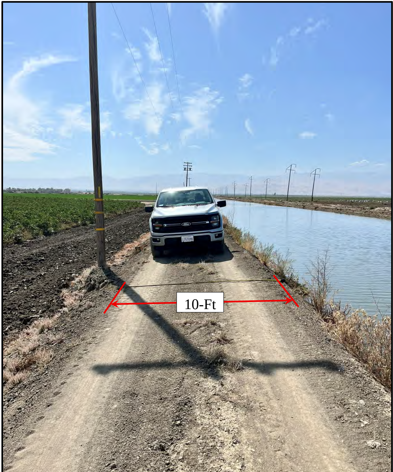
Looking south at the southern end of bank rebuild project proposed for 2026.
