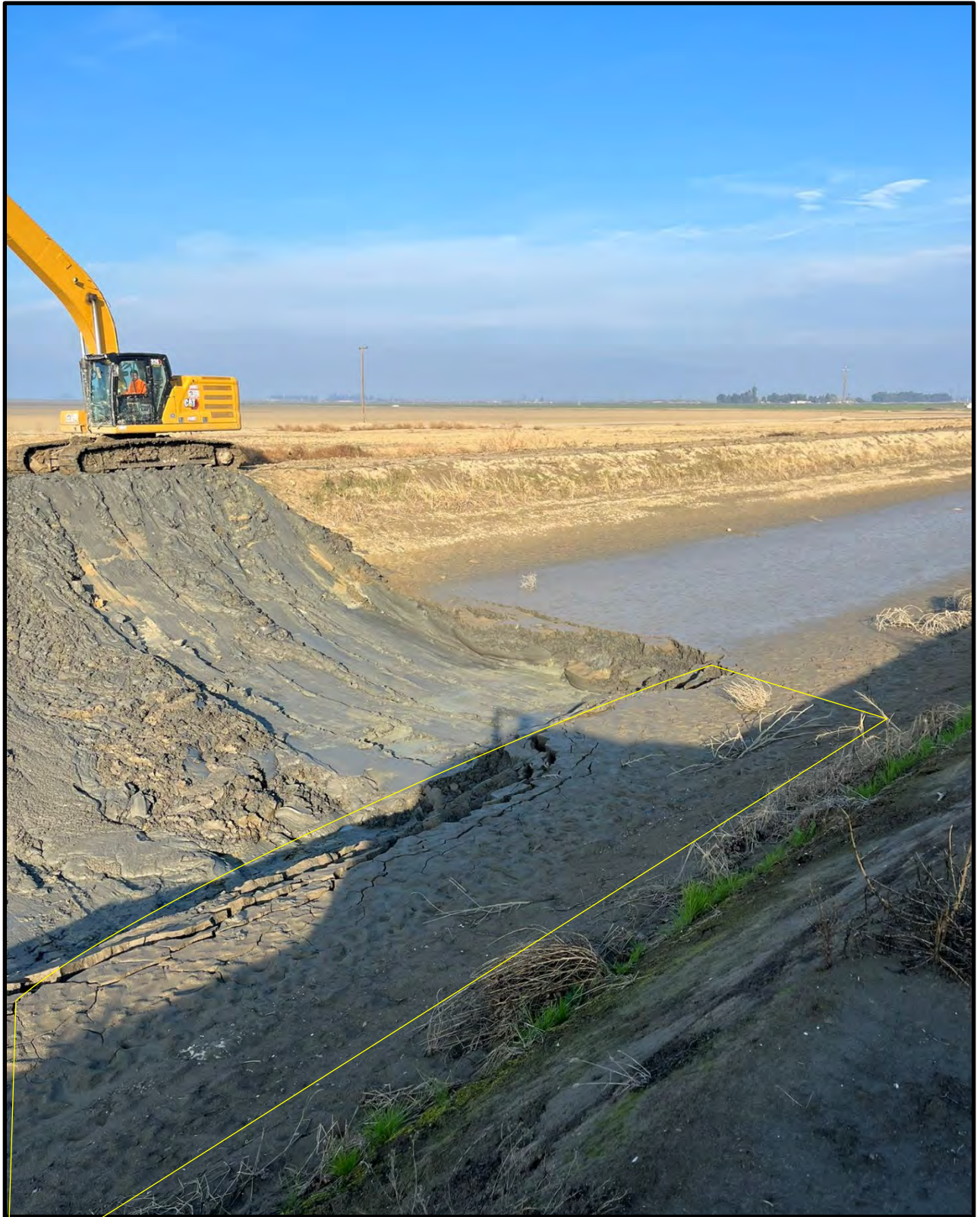
2023 Rim Ditch dredging. Note bench left behind.
