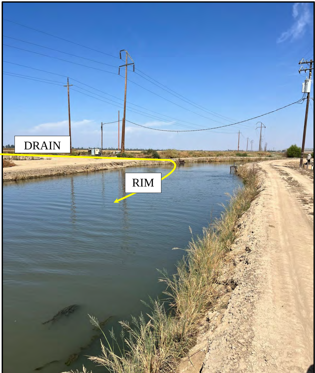
Looking north at the northern end of bank rebuild project proposed for 2026.
