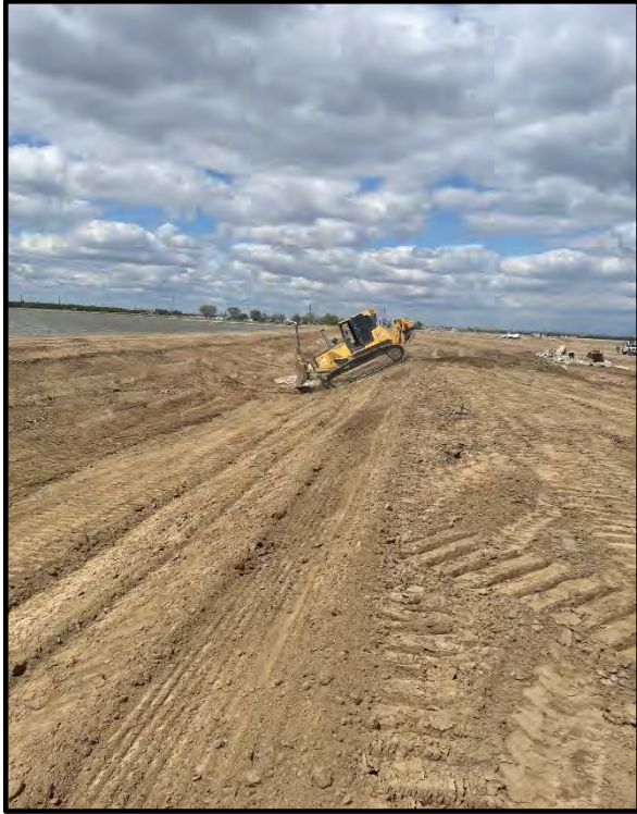
Photo 51: Canal improvement south of weir, looking north.
