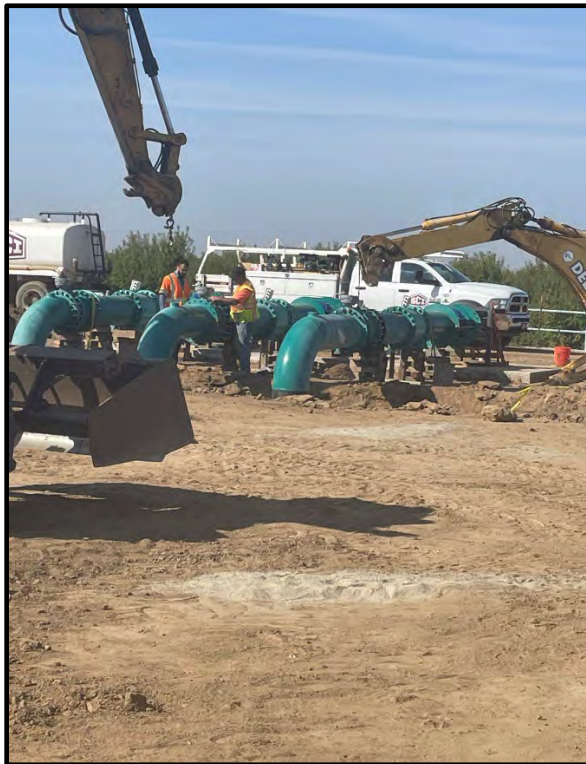
Photo 65: Pump discharge construction complete.
