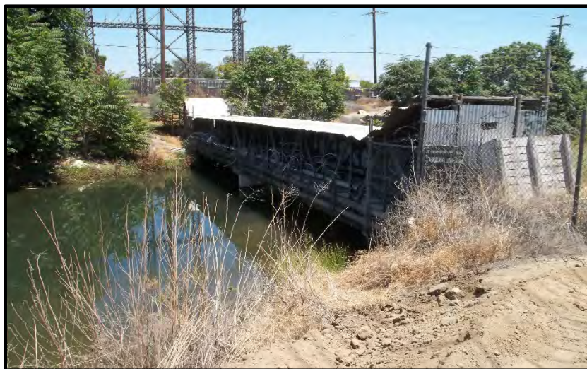
Photo 1: PG&E utility bridge, circa 2013
