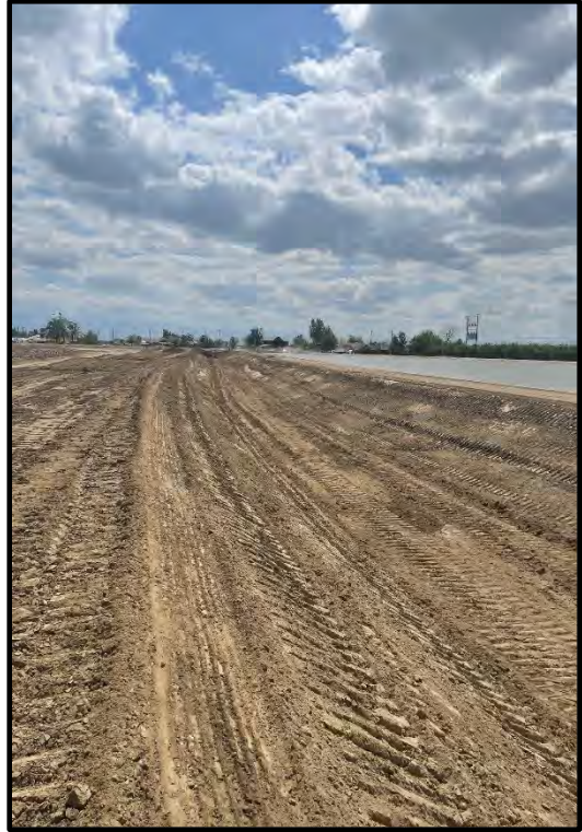
Photo 52: Canal improvement south of weir, looking south.
