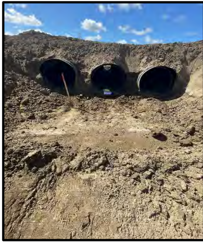
Photo 47: Road crossing culvert, looking south.
