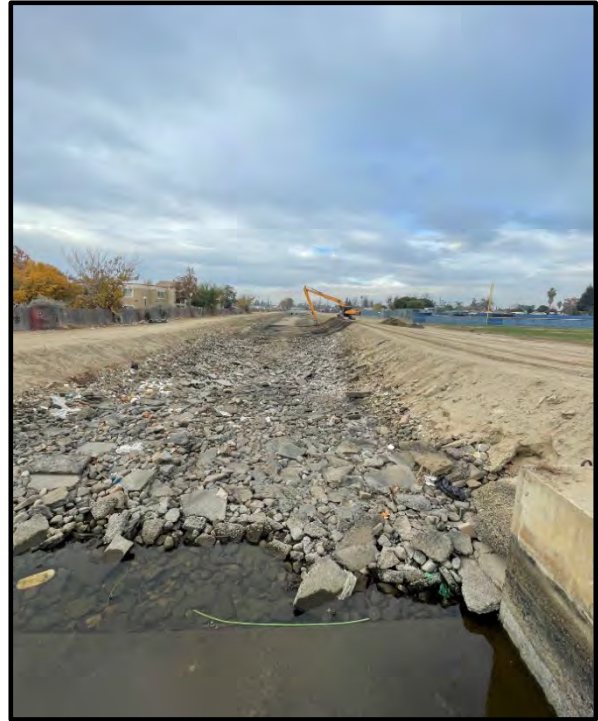
Photo 30: Central Branch, looking north from Brundage Lane
