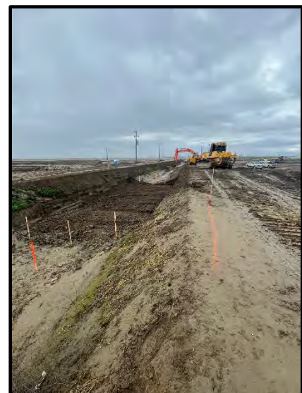
Photo 46: Preparation for road crossing.
