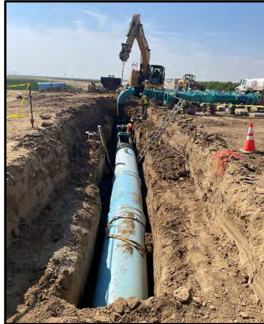
Photo 64: Pump discharge tie-in to 36" main line.
