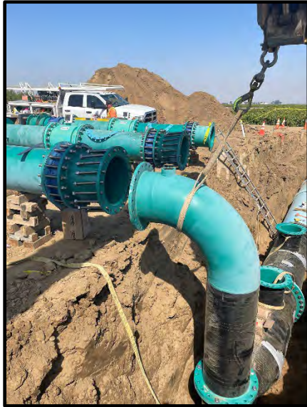
Photo 63: Pump discharge construction.
