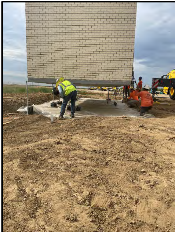
Photo 58: Setting Pump House.
