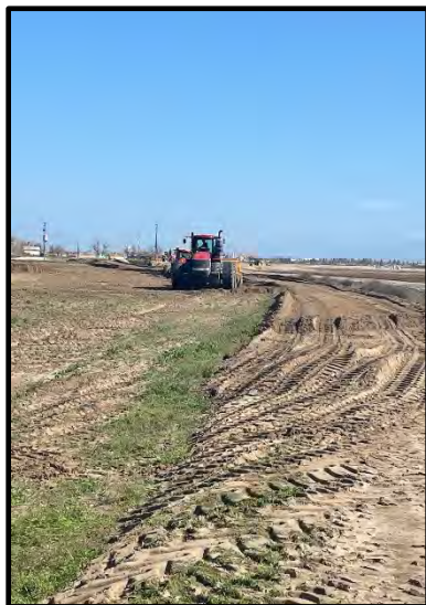
Photo 45: Pond 4 construction, looking north.
