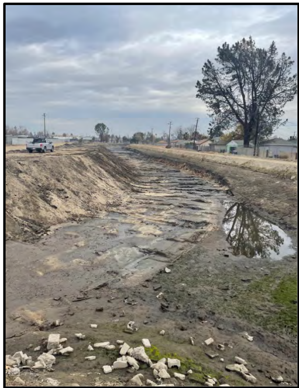
Photo 28: Kern Island, looking north from KI/Central split weir
