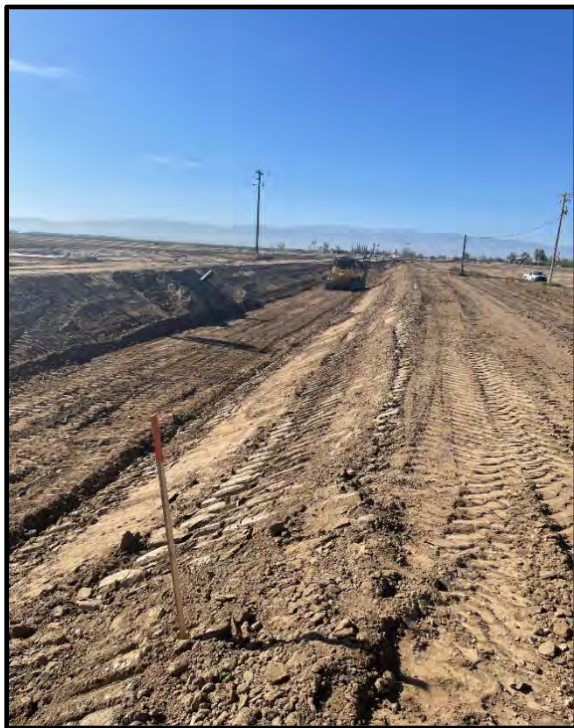
Photo 49: Canal improvement. North of weir.
