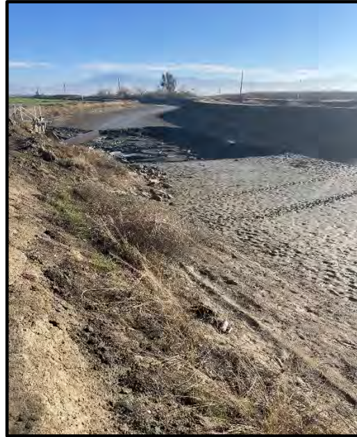
Photo 34: Rim Ditch, looking east.
