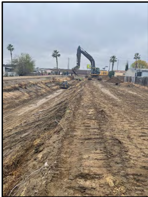
Photo 31: Branch Once Canal, look south from White Lane
