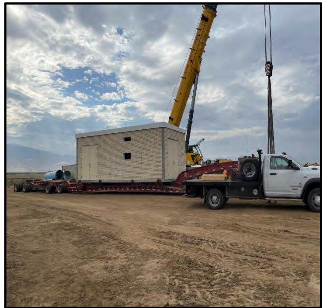
Photo 57: Pump House arrives on site.
