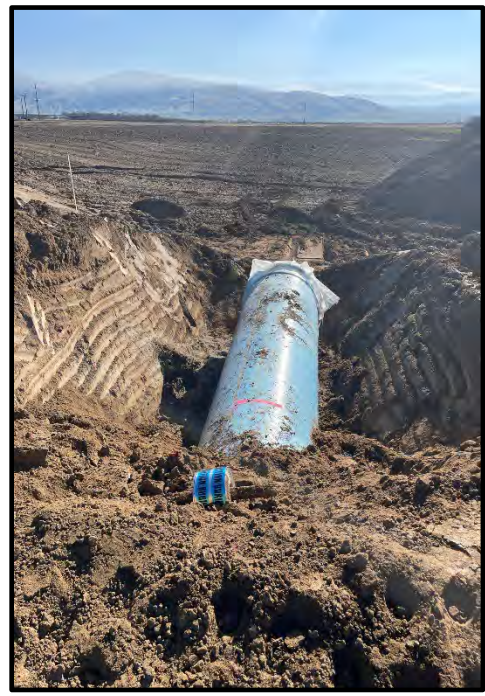
Photo 55: Discharge into Pond 1
