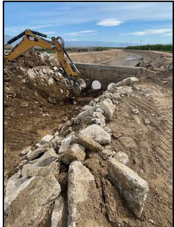
Photo 41: Rip-rap installed, looking south.
