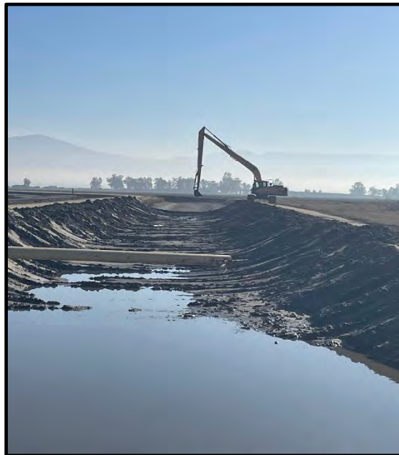
Photo 35: Rim Ditch, looking east
