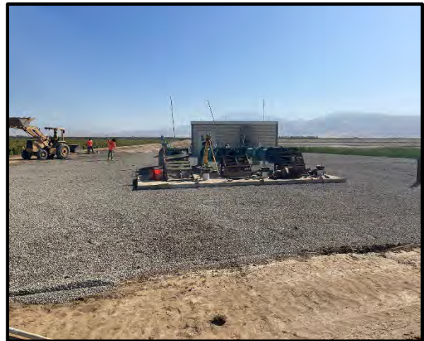
Photo 66: Pump site gravel installation.
