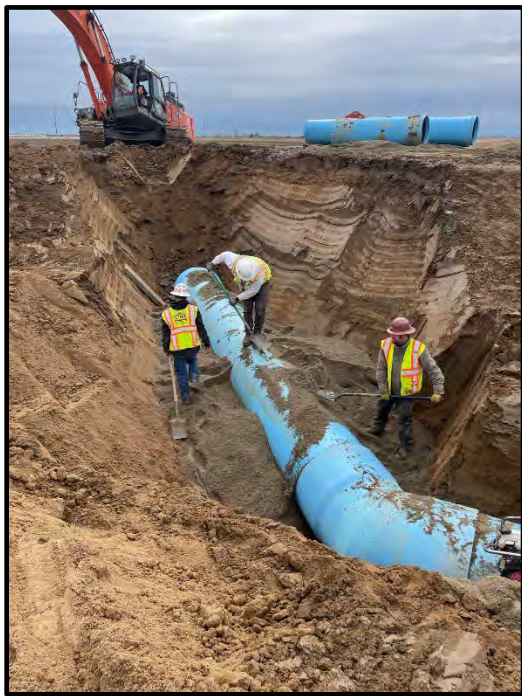
Photo 54: Installation of discharge into Pond 1
