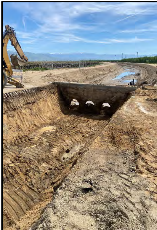
Photo 40: Crossing removed, canal shaped, looking south.
