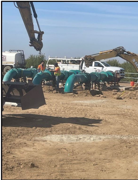
Photo 65: Pump discharge construction complete.
