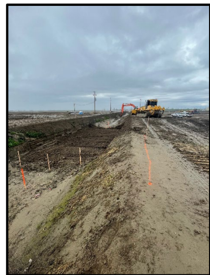
Photo 46: Preparation for road crossing.
