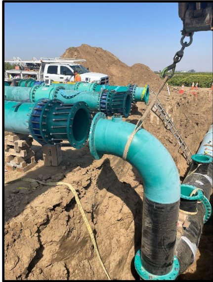
Photo 63: Pump discharge construction.
