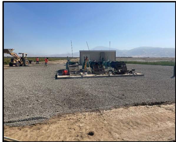
Photo 66: Pump site gravel installation.
