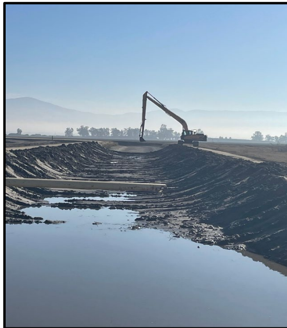
Photo 35: Rim Ditch, looking east
