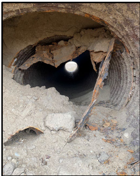
Photo 36: Center culvert pipe, looking north.
