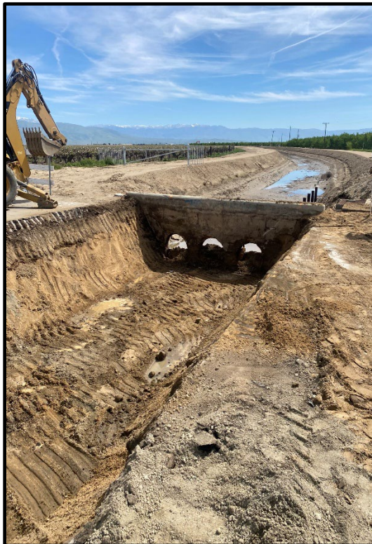
Photo 40: Crossing removed, canal shaped, looking south.
