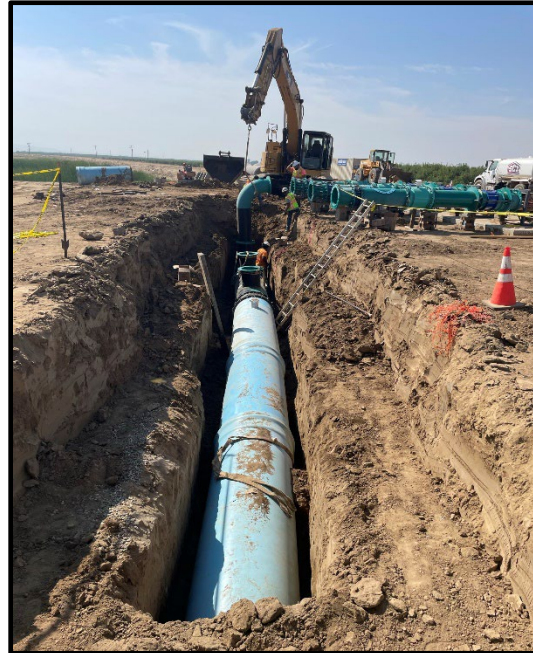
Photo 64: Pump discharge tie-in to 36" main line.
