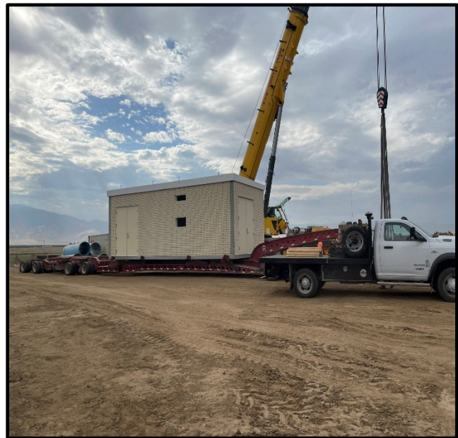
Photo 57: Pump House arrives on site.
