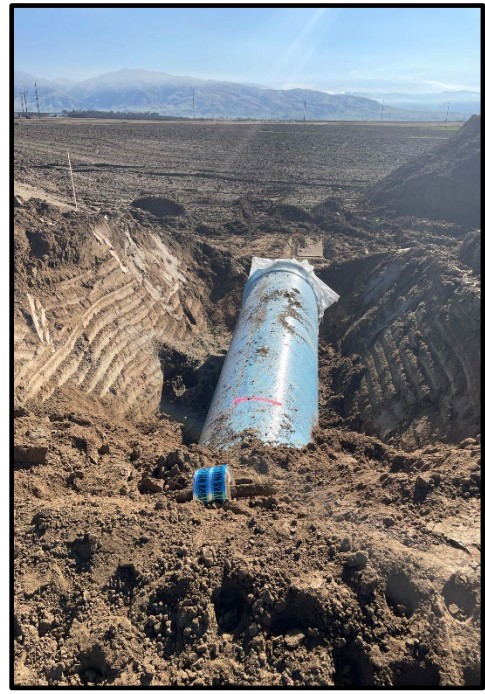
Photo 55: Discharge into Pond 1
