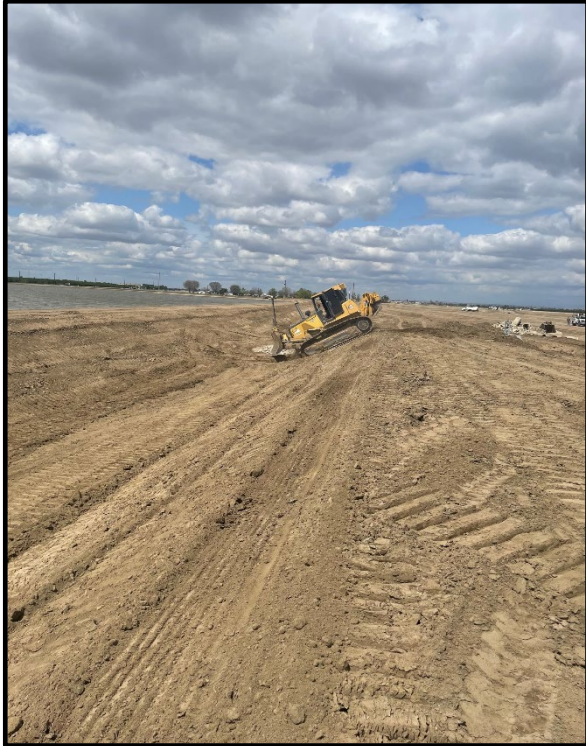
Photo 51: Canal improvement south of weir, looking north.
