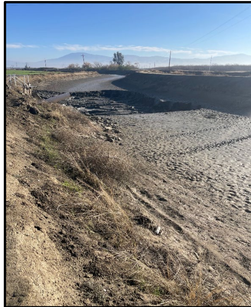
Photo 34: Rim Ditch, looking east.
