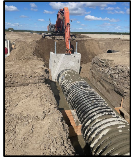
Photo 48: Inlet to Pond 1
