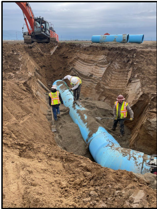
Photo 54: Installation of discharge into Pond 1
