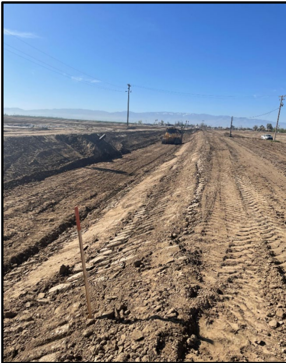
Photo 49: Canal improvement, North of weir.
