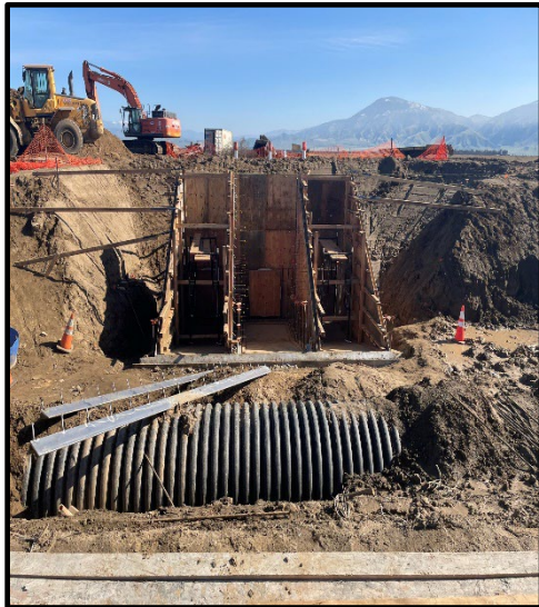
Photo 56: Pump inlet construction.
