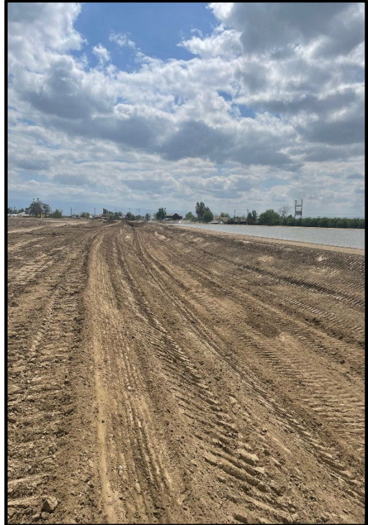
Photo 52: Canal improvement south of weir, looking south.
