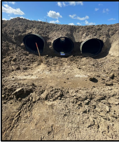
Photo 47: Road crossing culvert, looking south.
