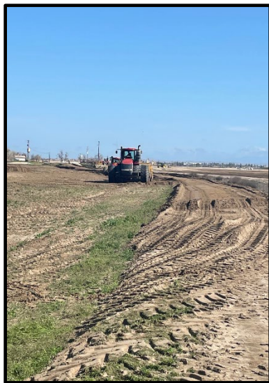
Photo 45: Pond 4 construction, looking north.
