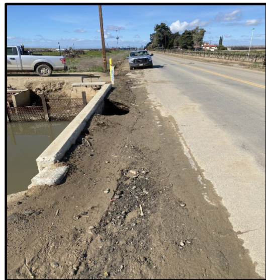
Photo 37: Eastside Canal crossing at Buena Vista Blvd, looking east.
