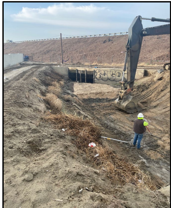
Photo 32: Branch One Canal, looking southwest towards Highway 99
