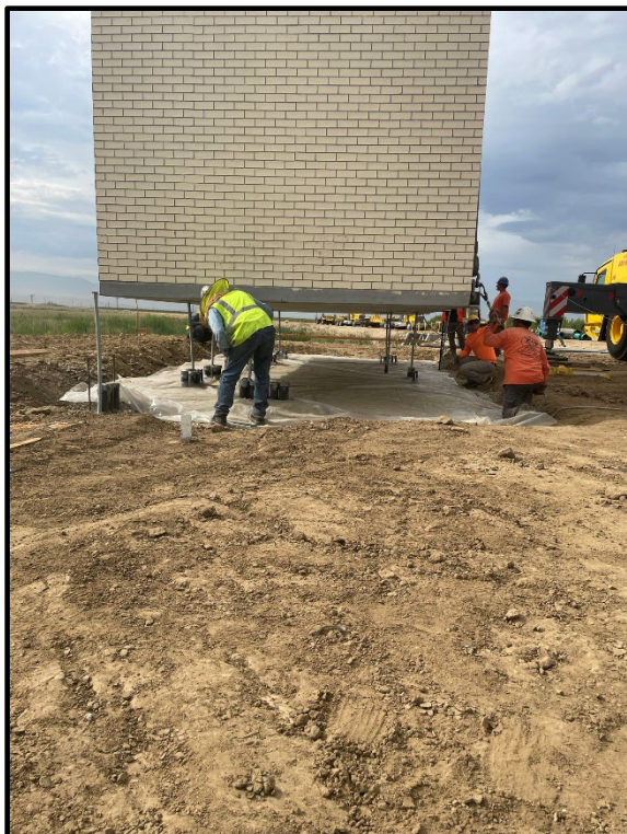
Photo 58: Setting Pump House.
