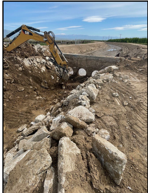
Photo 41: Rip-rap installed, looking south.
