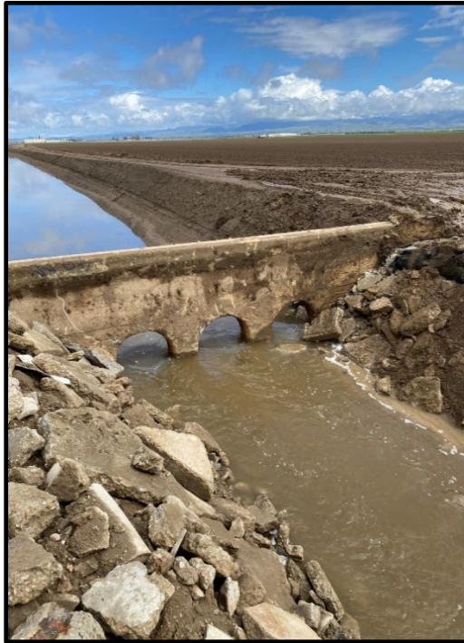
Photo 42: Eastside Canal flowing again, looking north.
