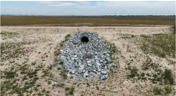
Pond 3 Turnout outlet.
