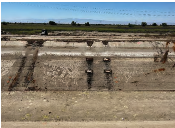
Siphon pipe demolition completed.
