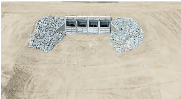
North Pioneer turnout completed.
