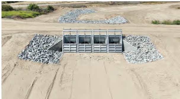
Basin 11 turnout completed.
