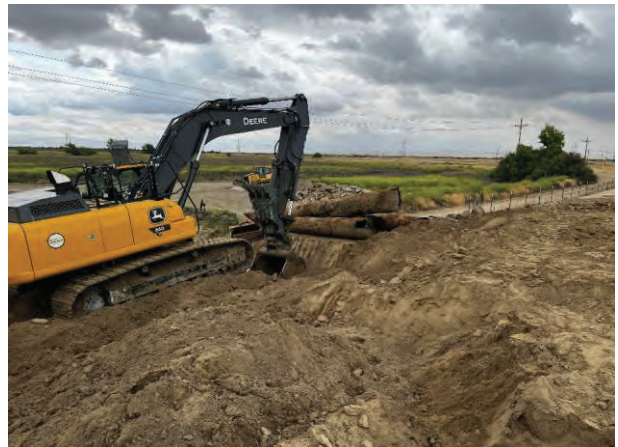
Siphon demolition and site preparation for cofferdam installation.
