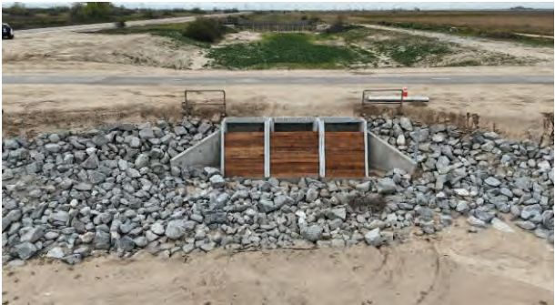
Basin 9 Turnout inlet.
