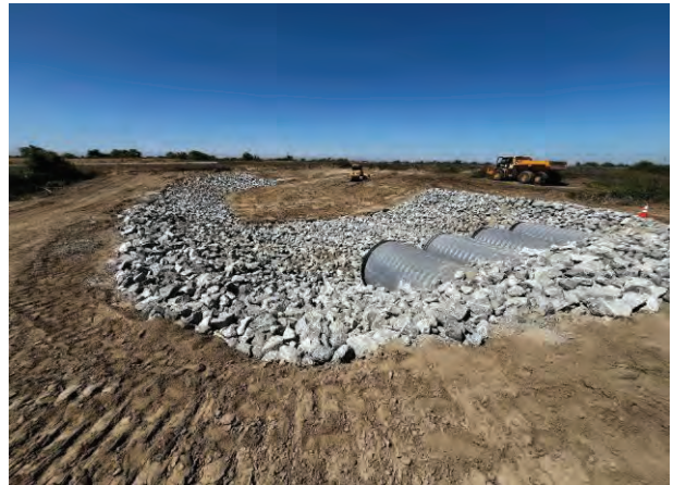
Basin 11 turnout outlet piping and rock slope protection.
