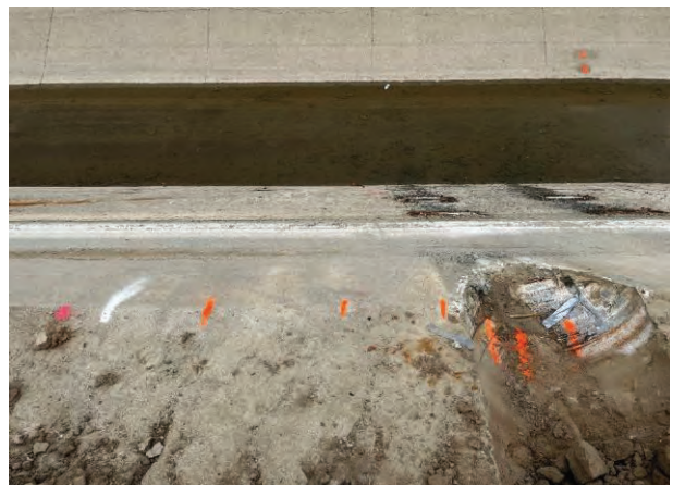
Layout on liner for cofferdam installation.
