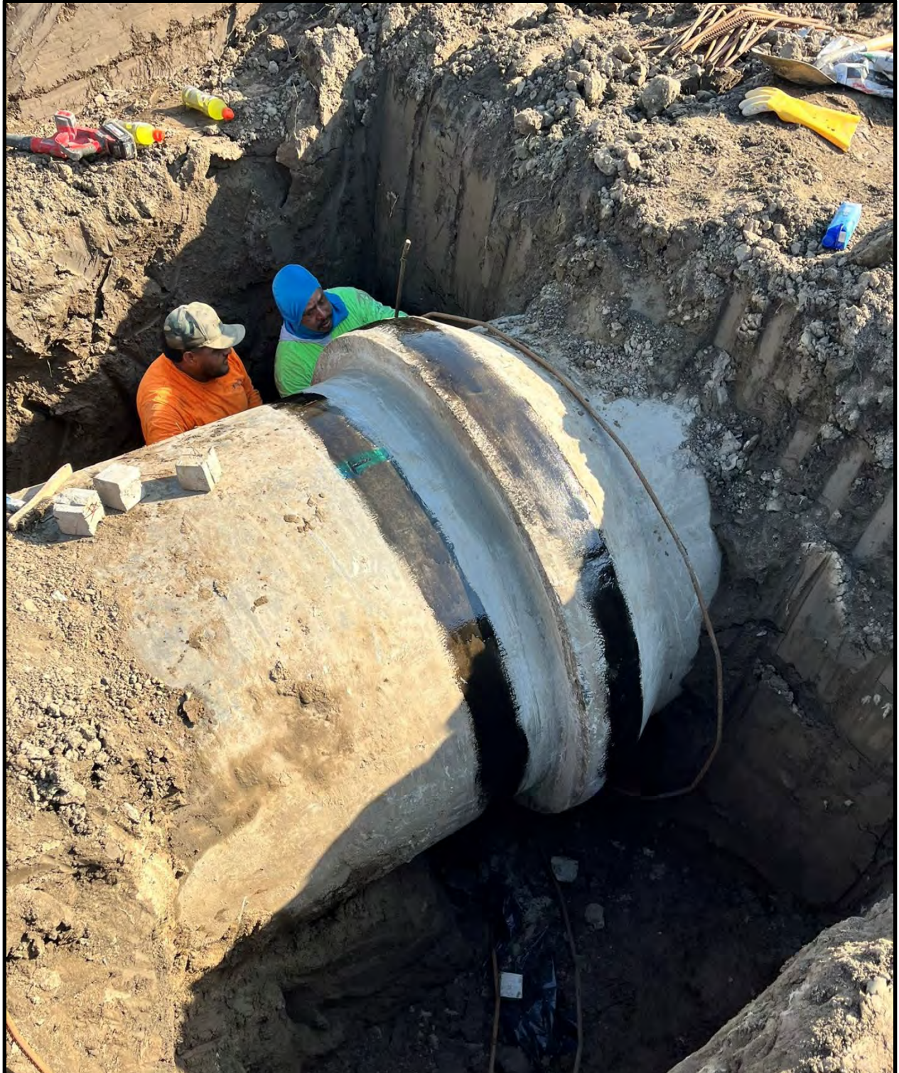
Photo showing the Swellstop adhesive/primer and Elephant Armor joint sealant.
