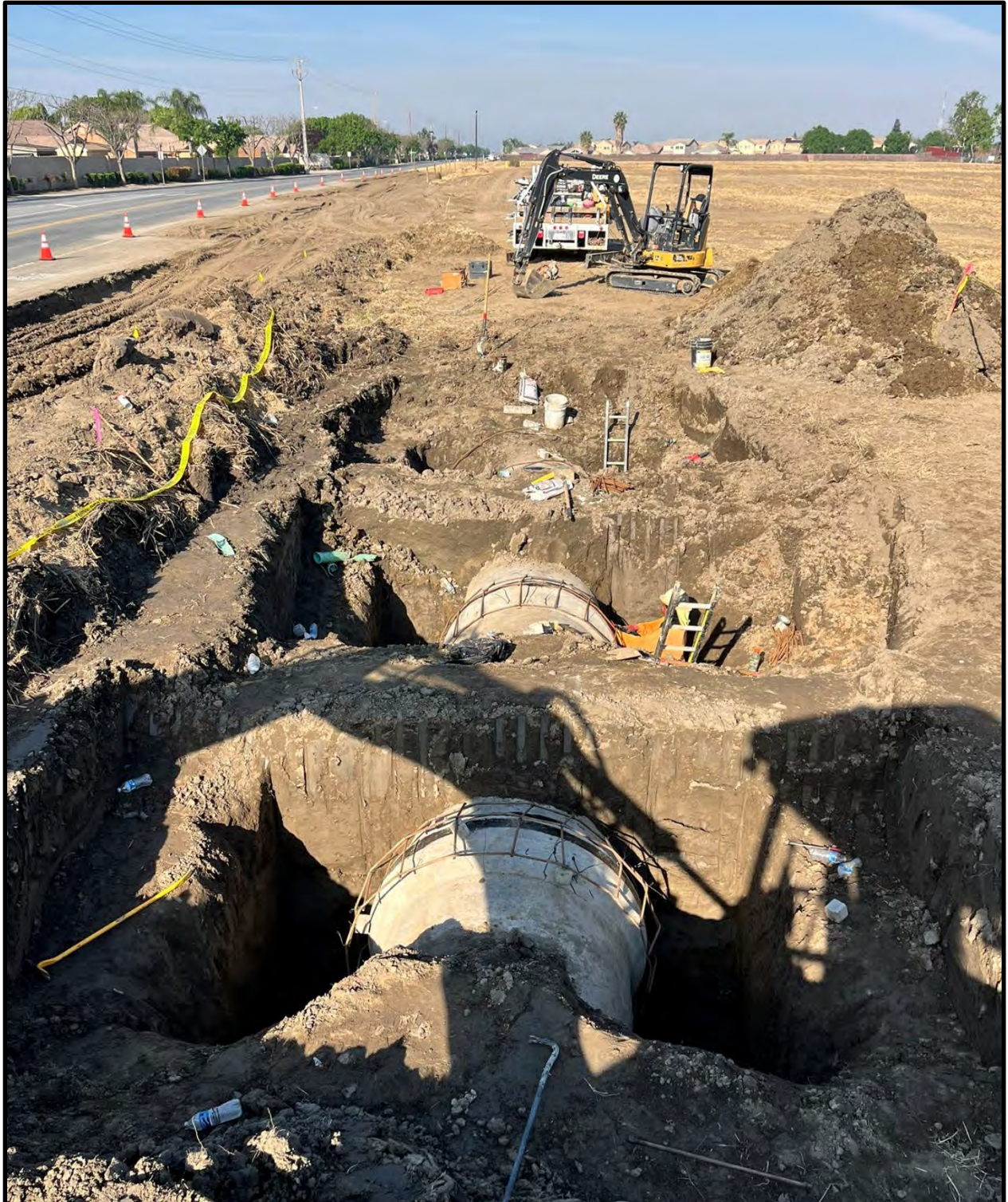
Looking west at three exposed joints of the Hirshfield pipeline.
