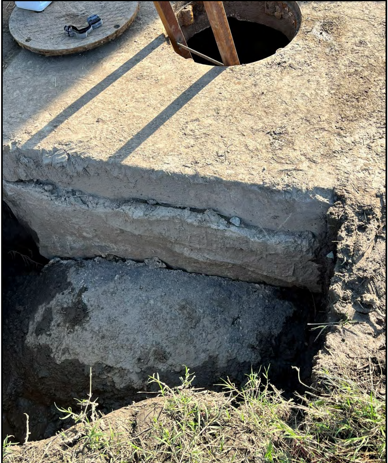
Showing the Hirshfield pipeline entering the west side of the manhole.
