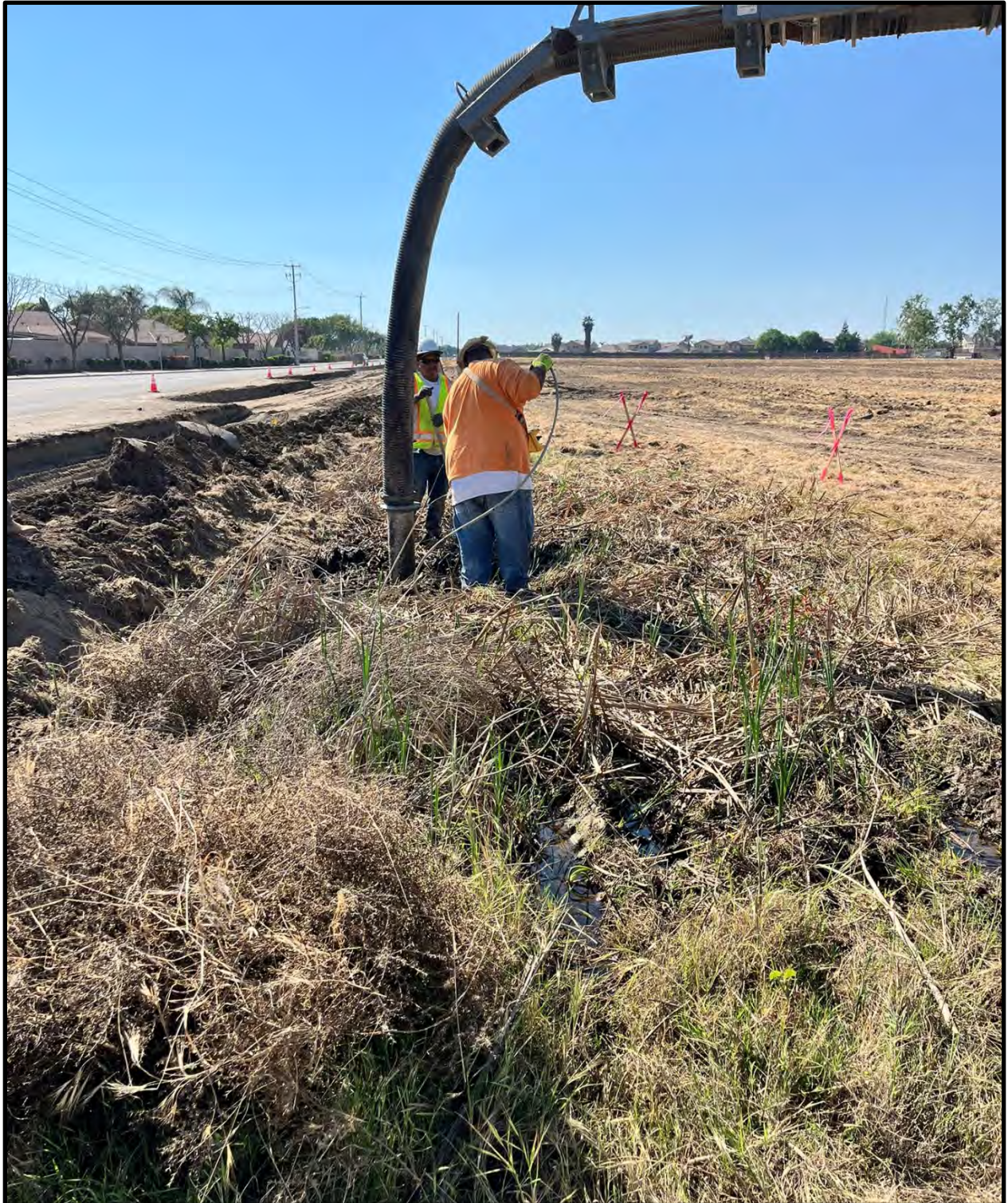
Looking west at hydrovac exposing the Hirshfield pipeline.
