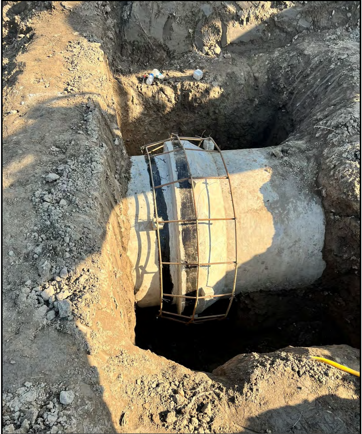
Photo showing a completed rebar cage for the field collar
