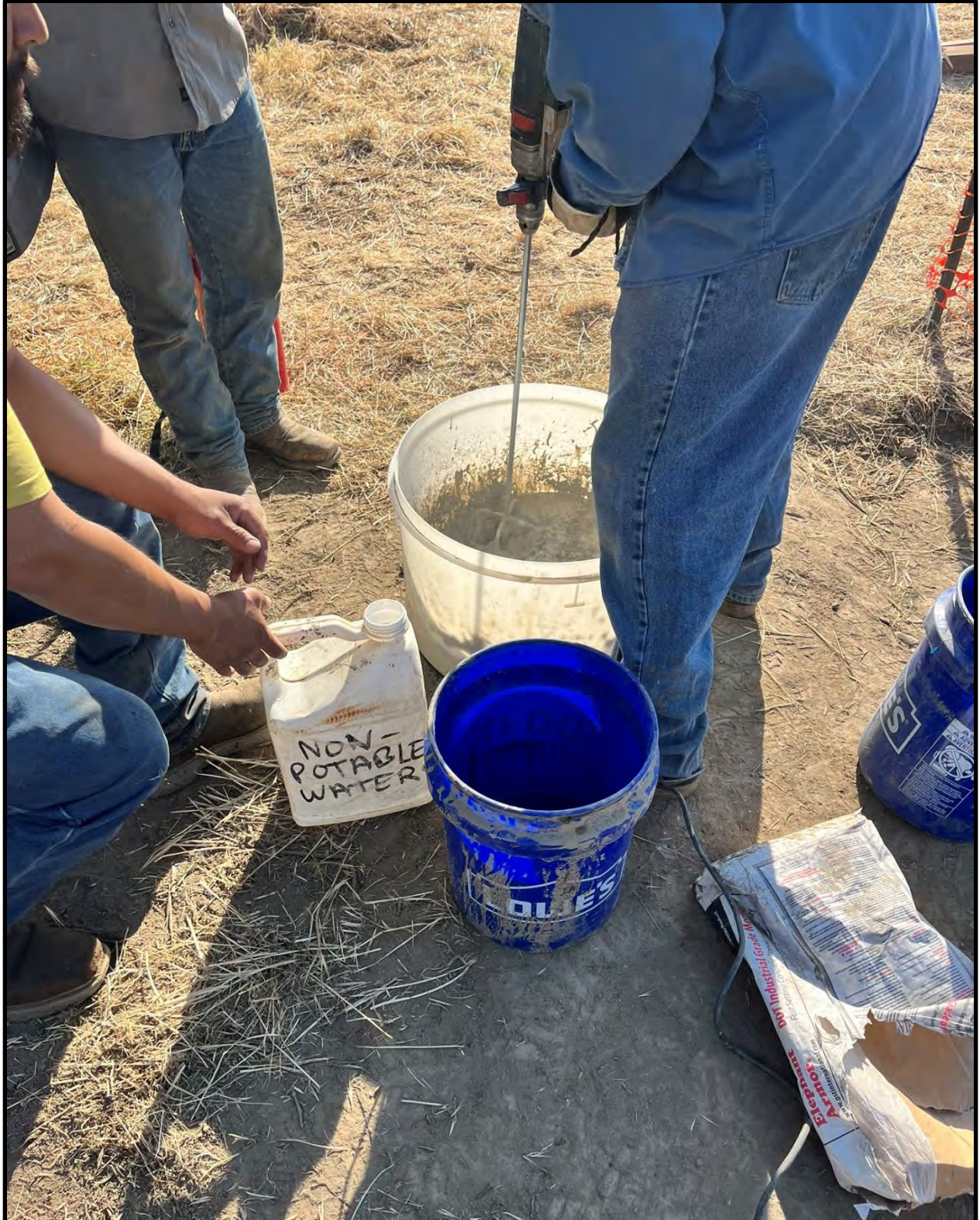
District staff mixing the Elephant Armor sealant.
