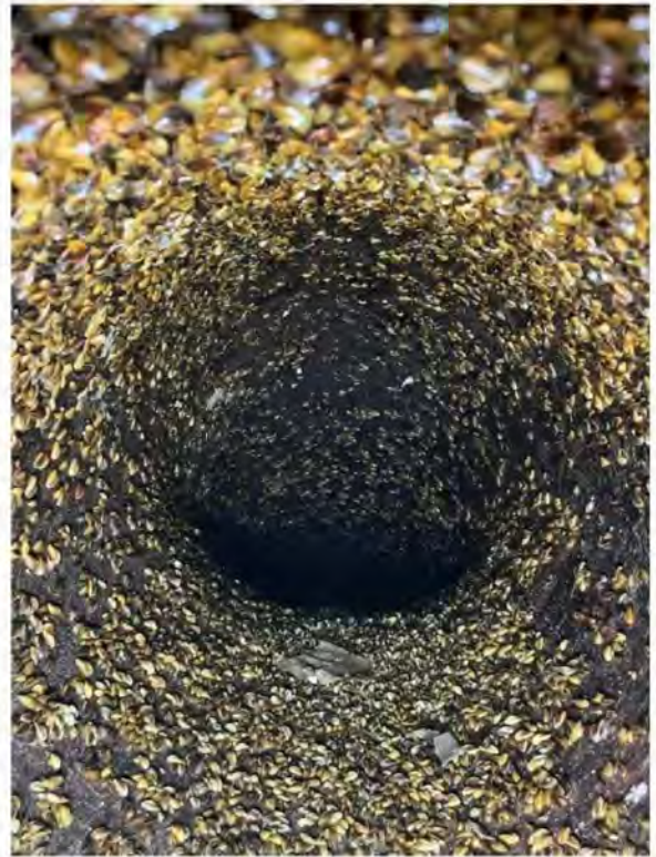
Golden mussels colonizing the inside of a water pipe. SOURCE: Presentation by Arvin-Edison Water Storage District
