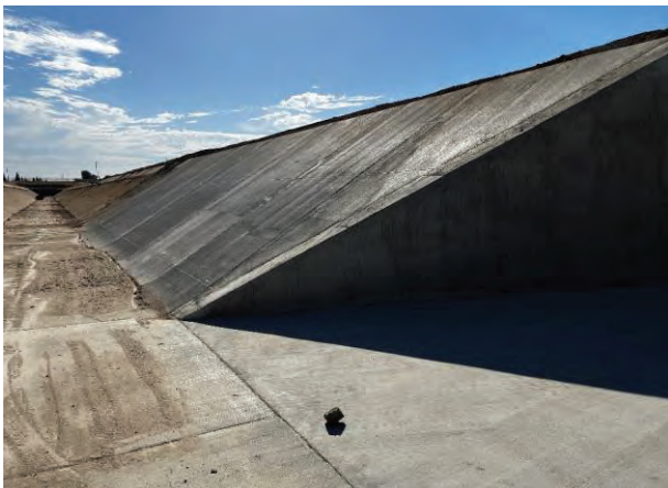
Liner panels replaced.
