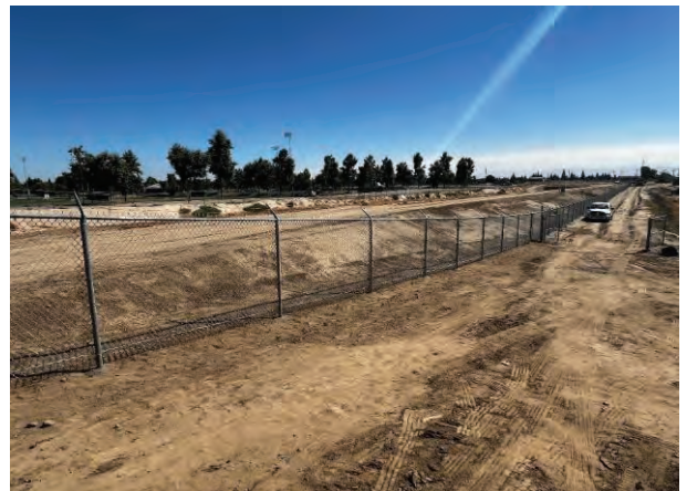
Fencing replaced and ID1 levee restored.
