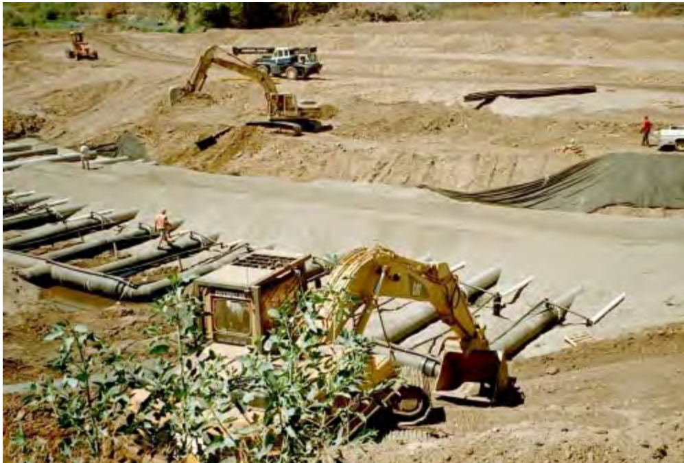
A grid of percolation pipes create an infiltration gallery in the bed of the Tuolumne River in 2001. Photo: Turlock Irrigation District.
