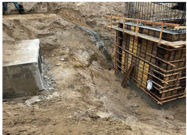
Pioneer Canal box culvert sawcut.
