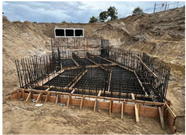
Structure slab rebar installed.
