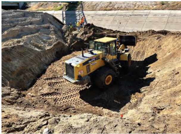
Existing structure demoed and foundation compacted.
