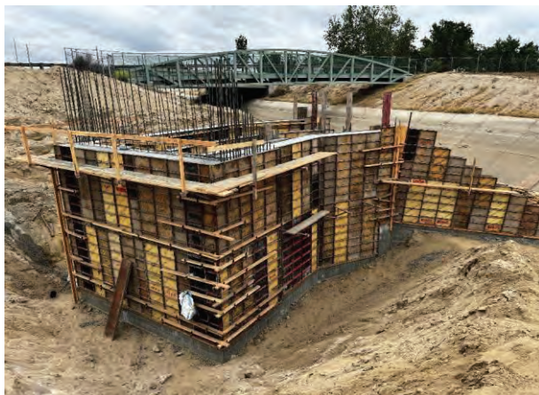
Concrete walls placed.
