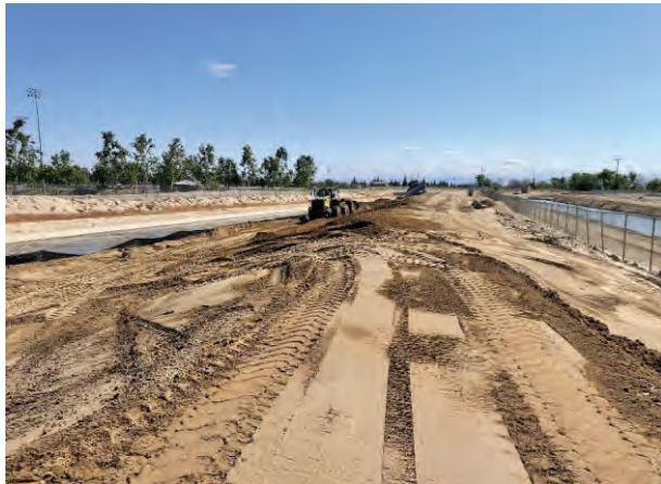
Removing plates from shoring system.
