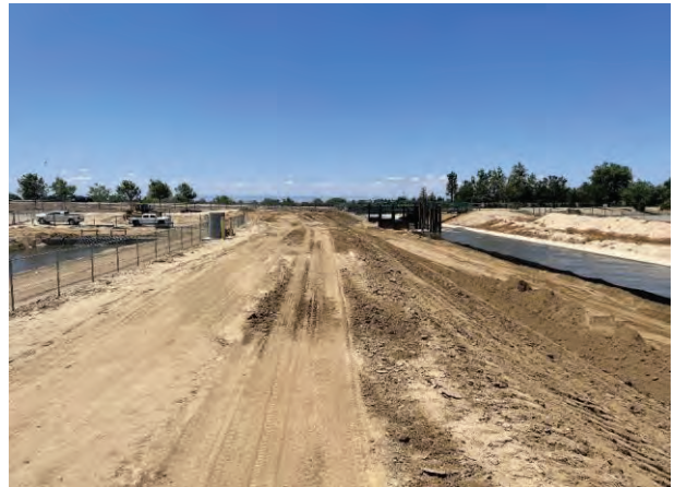
Plates within canal prism removed and slope armored with rip-rap.
